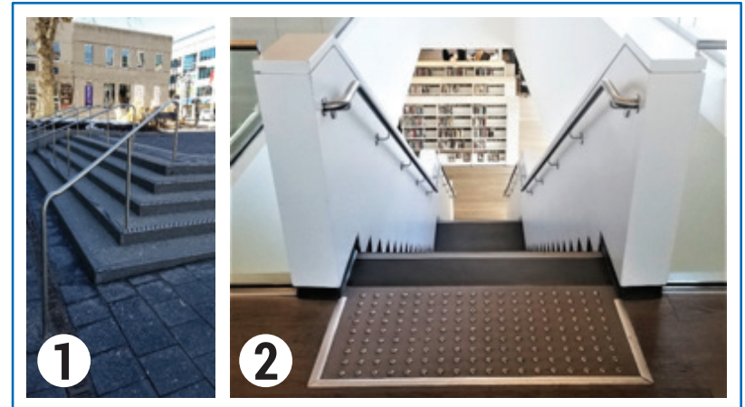
Photo 1. Stair surfaces that are stable, firm, slip-resistant, and non-glare (4.3.b)
