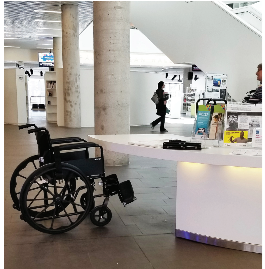
A lowered accessible counter surface (6.5.2.c) providing adequate space for knees (6.5.2.d) (Image: Cities and Environment Unit)
