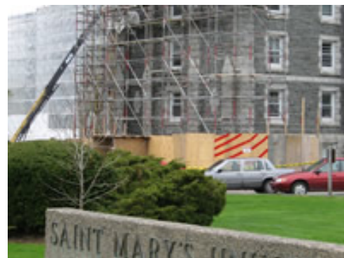
Stonework repairs are carried out on the McNally building
